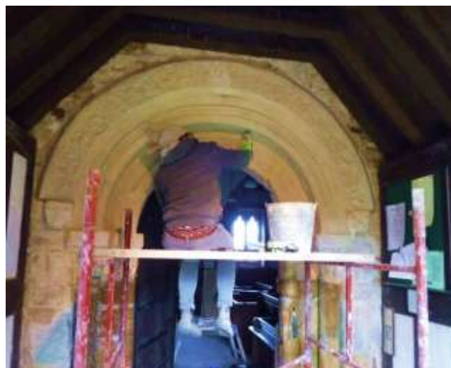
Repairing the arch at All Saints Church
